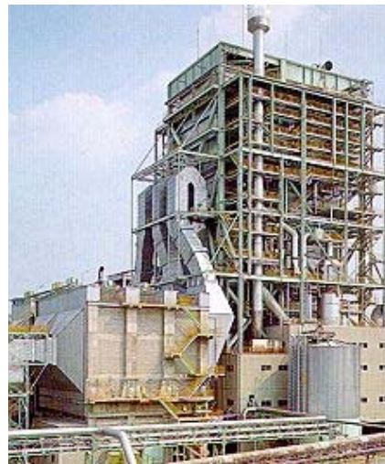
Black liquor recovery boiler (in colder climates it may be enclosed)
